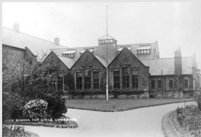
©Windows on Warwickshire
