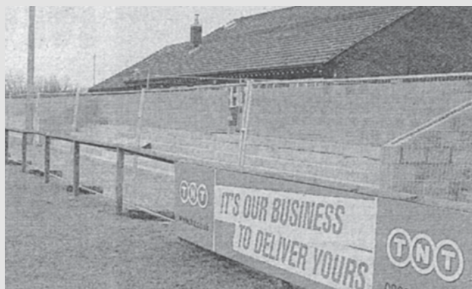
The standing terrace takes shape in front of the Nuns clubhouse.
